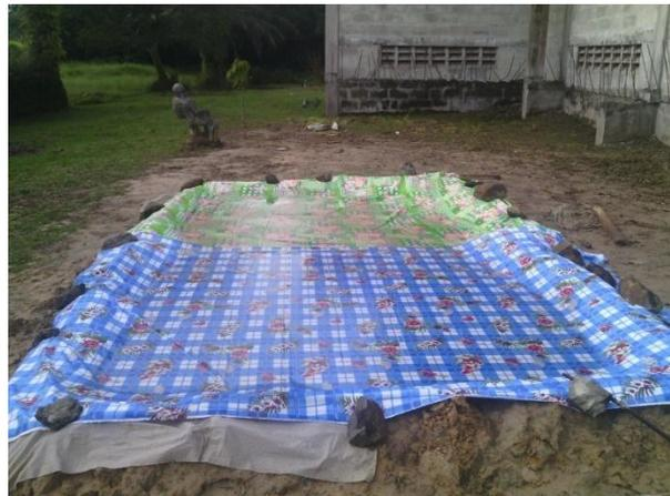
Fig. 11: Clay trough filled with slip covered with cotton based spread sheets set and left to dry
