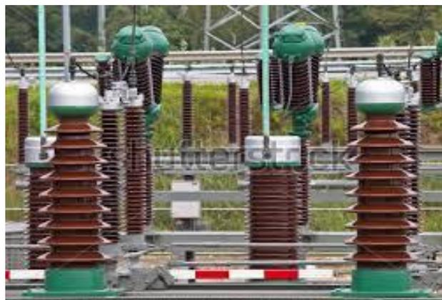
**Plate vii: Electric insulators manufactured from ceramic materials**
