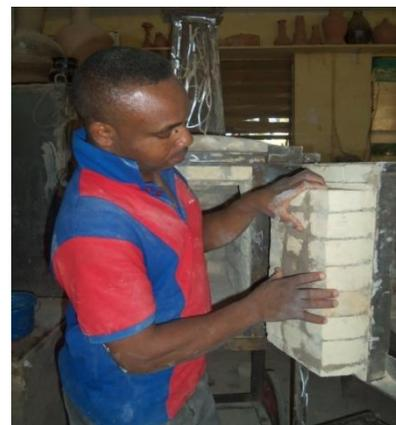
Fig. 11: Constructing the kiln
